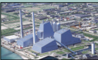
The worlds largest, the Energi E2 Avedøre pellet CHP plant, Denmark
