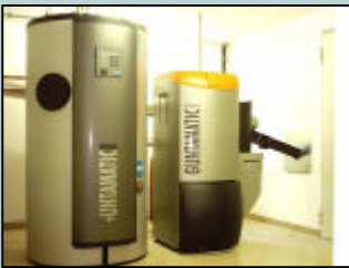
Modern European heating facility for domestic use of wood pellets
